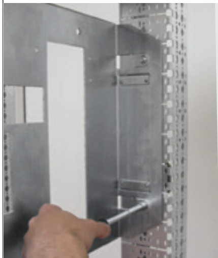
Locking the plate using M6 screws and clip-nuts
