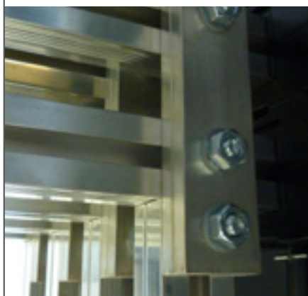
Connection between an aluminium busbar and a double main busbar created using aluminium bars
