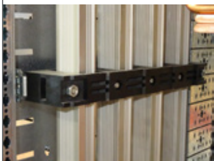
Position the busbars and tighten the supports to ensure the bars are held in place. (Tightening torque: see page 27)
