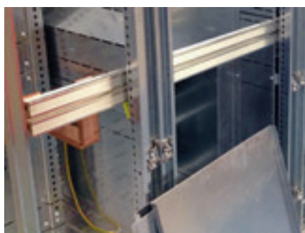
Main terminal consisting of a copper or aluminium bar
