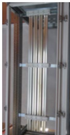
Fix the intermediate supports Cat.No 4 044 61 complying with the maximum distances.
