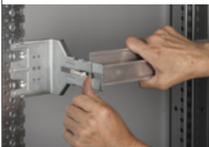
2 - Clipping the rail onto the attachment pieces (2 positions)
