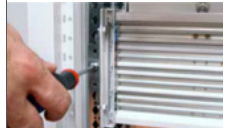
Position and fix the row distribution block on the functional uprights of the enclosure.
