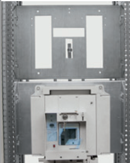
DPX 3 1600 supply inverter being mounted
